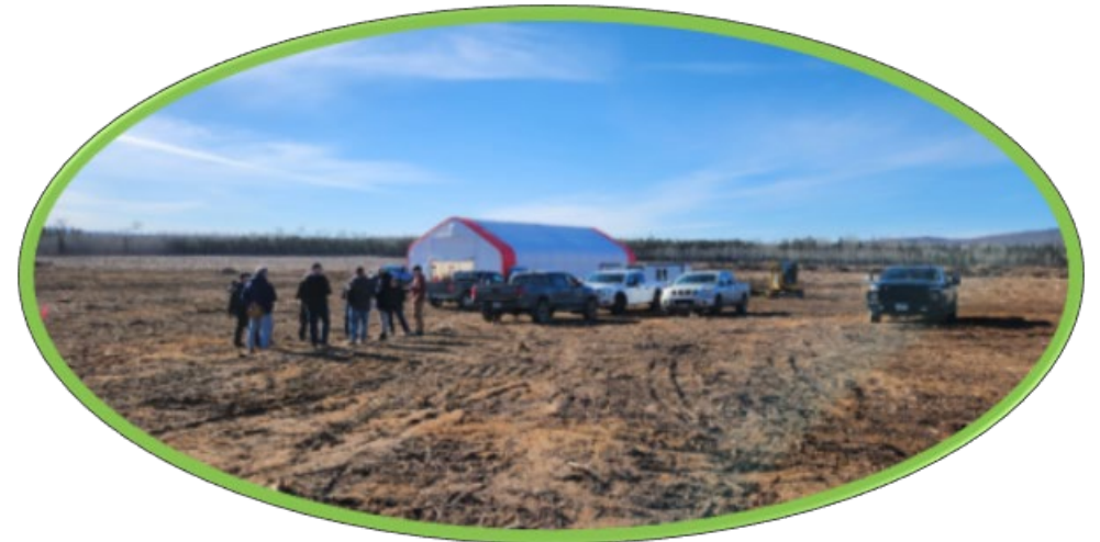
Lake Nipigon RNG and Biocoal Facility Site March 2024
